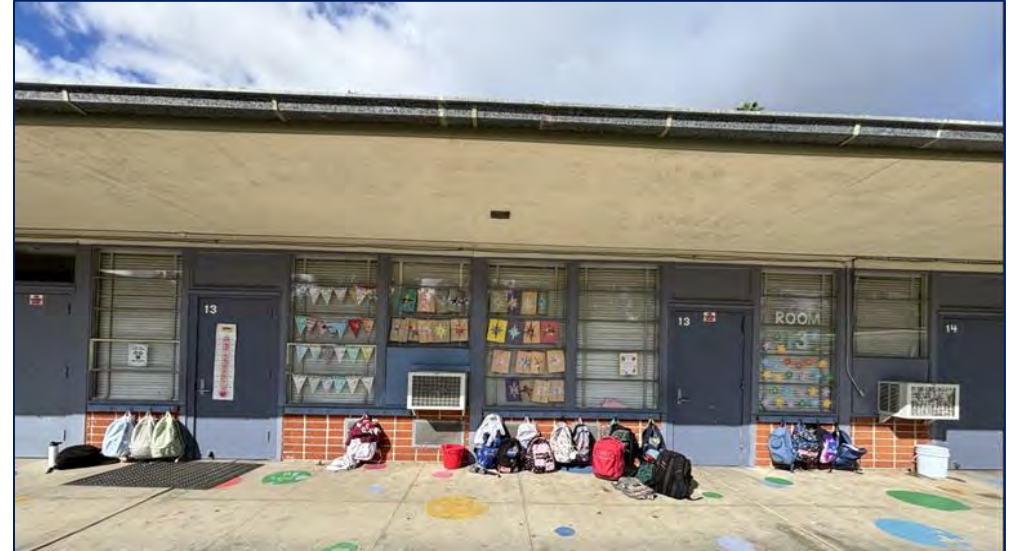
Typical Classroom Building with package wall units
