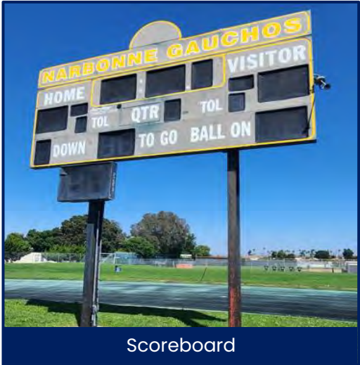
Area of Work
