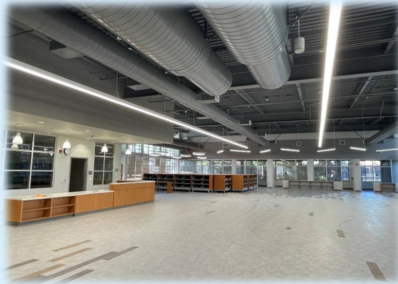
In Construction: Interior of Library
