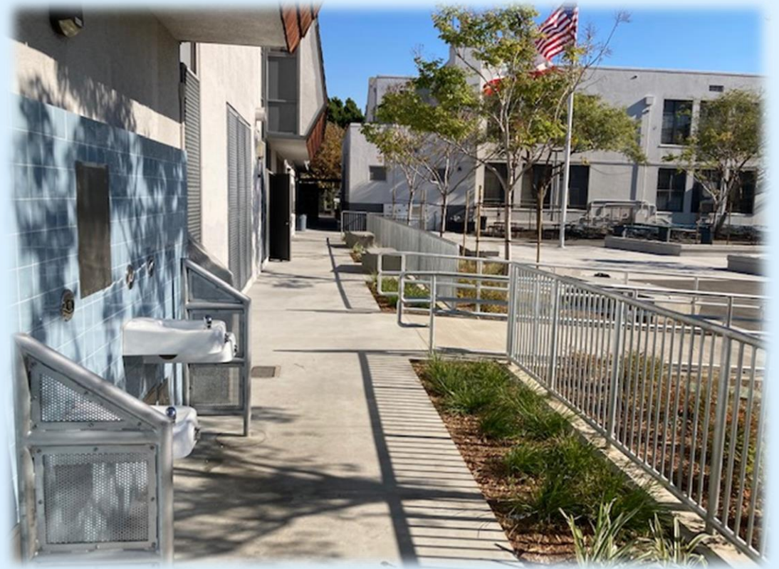
New Drinking Fountain and Walkway
