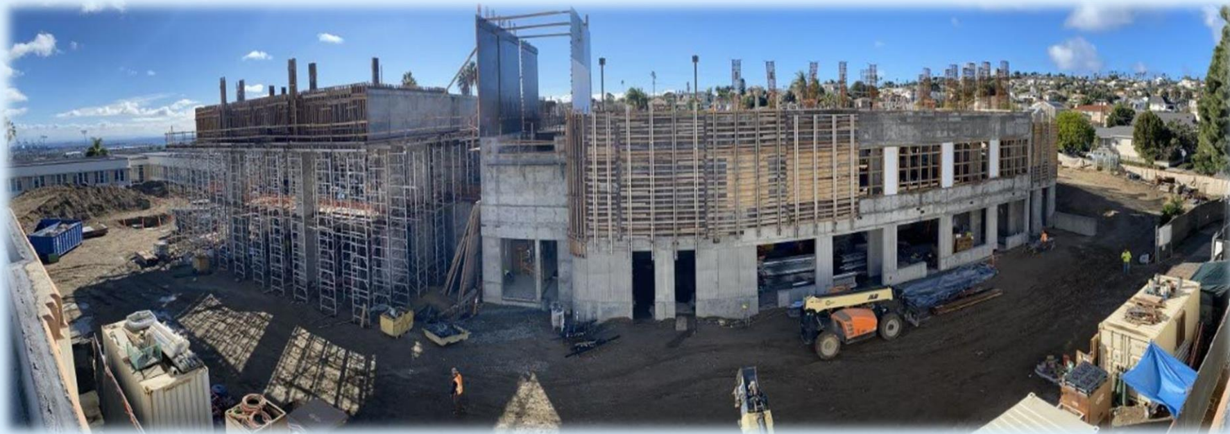
In Construction: Administration/Food Services/Classroom Building
