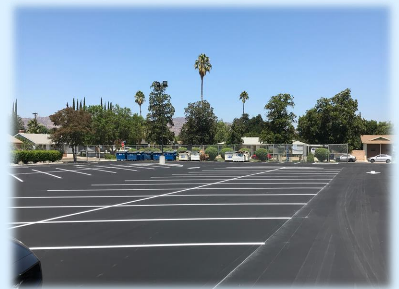
Freshly Paved Parking Lot
