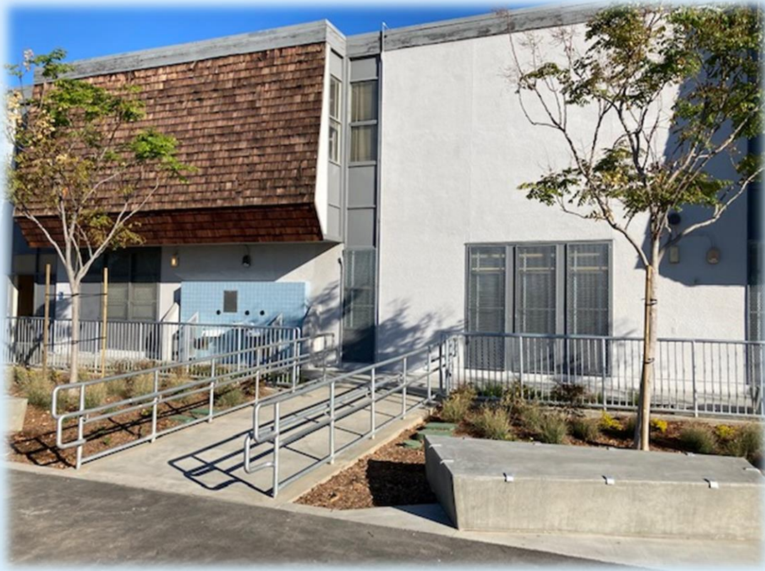
Accessible Handrail Ramp and Walkway
