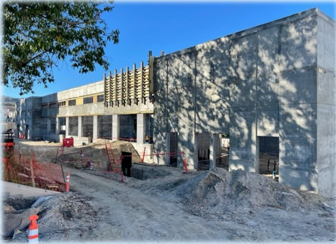
In Construction: New Visual Media/Band Building
