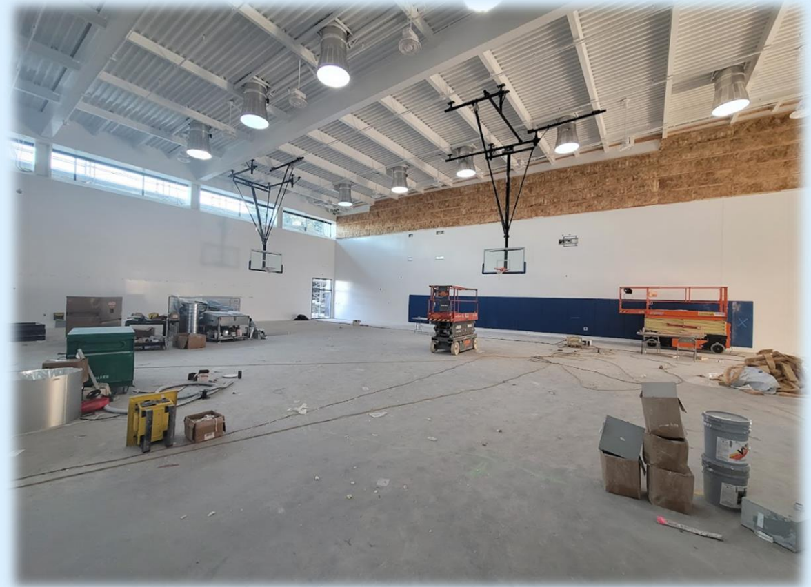
In Construction: New Gymnasium
