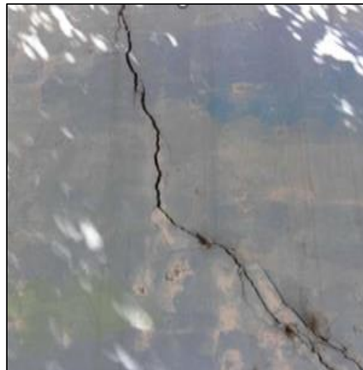
Cracked Retaining Wall
