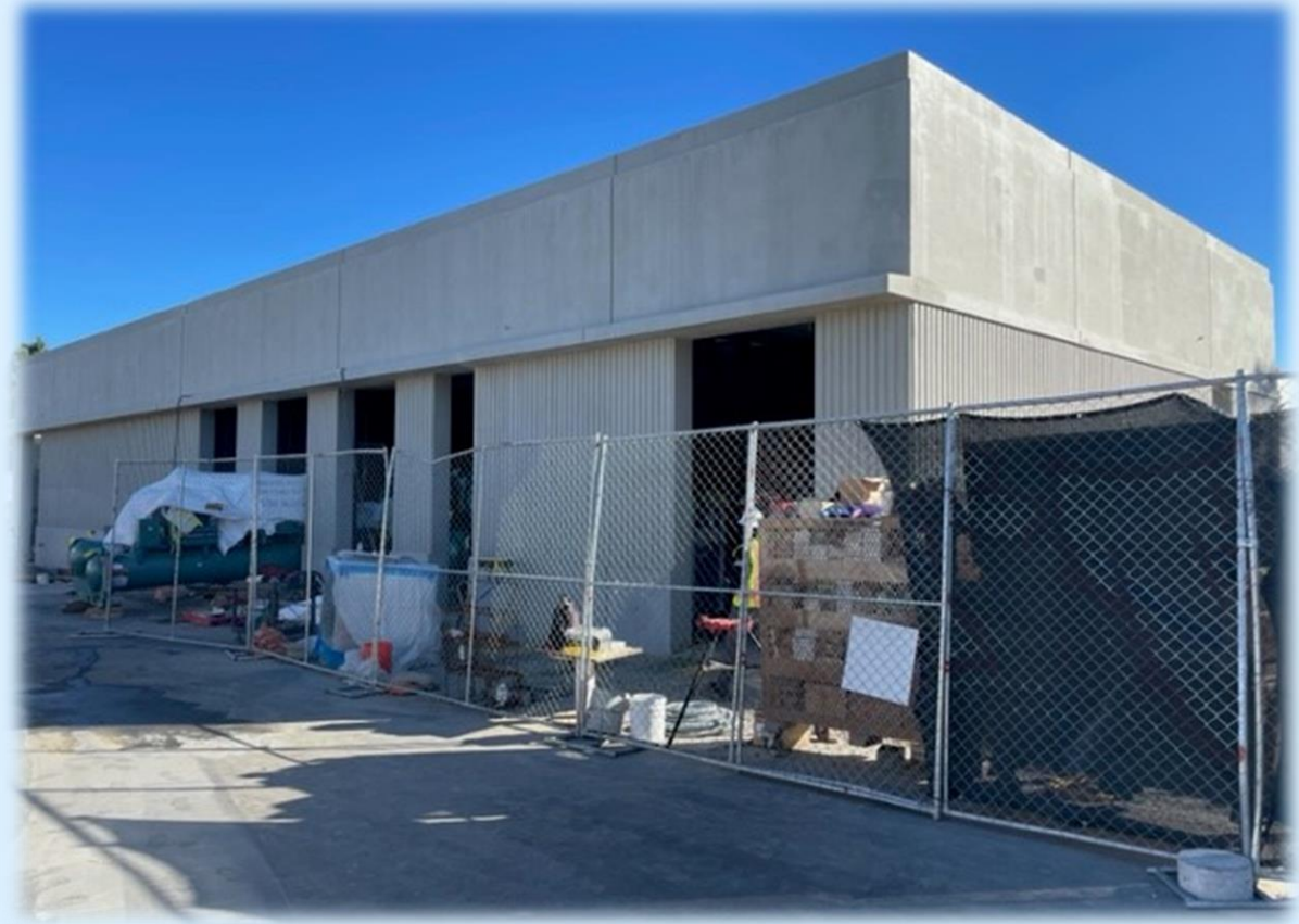
In Construction: New Central Plant Building
