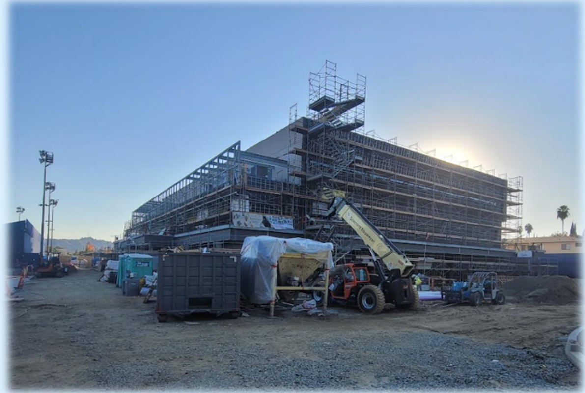
In Construction: Exterior of New Gymnasium
