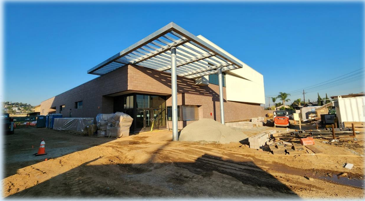
In Construction: New Gymnasium Building
