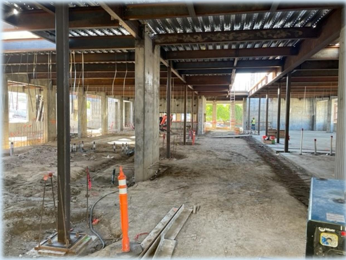
In Construction: Interior of New Administration Building
