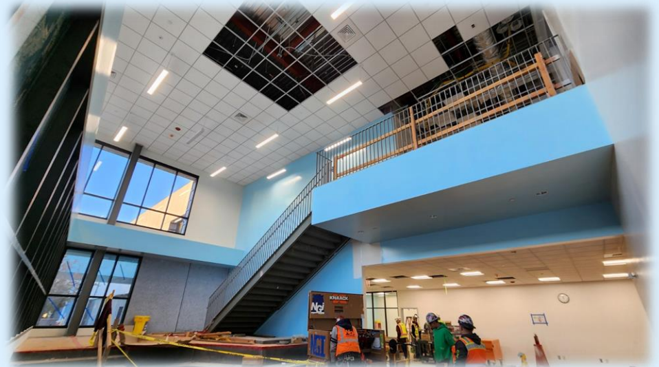
In Construction: Lobby
