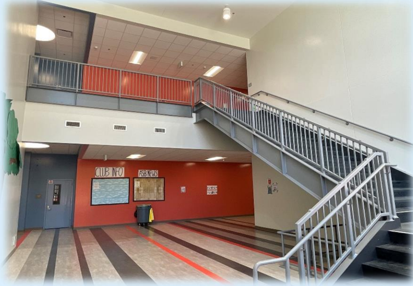
Completed: New Classroom Building
