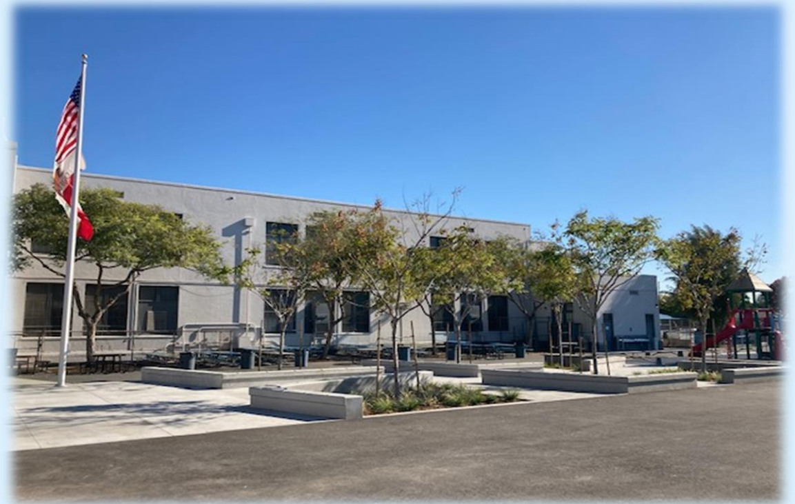
Flagpole and Concrete Landscaping Area
