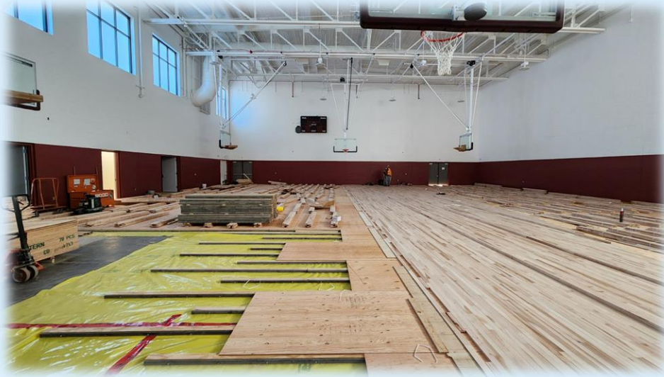
In Construction: Gymnasium
