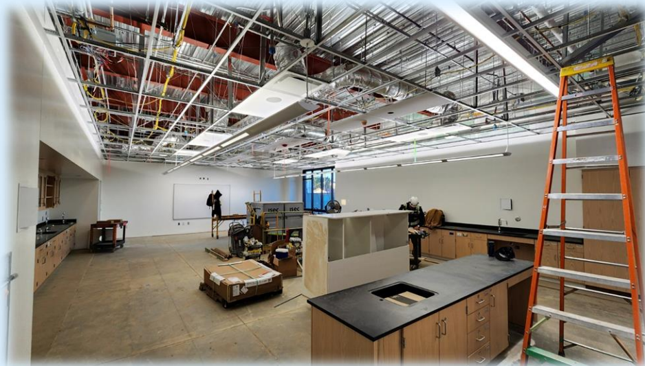
In Construction: Flex Science Room
