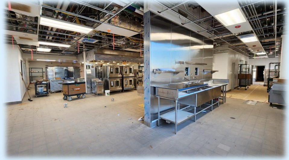
In Construction: Kitchen
