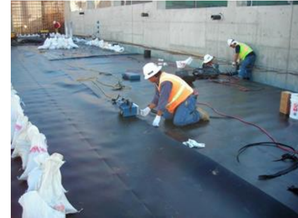
Installation of Membrane
