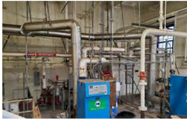
Photo 5: Existing boiler room
