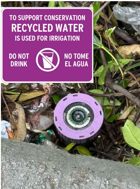
East Valley High School Recycled Water Irrigation installation – purple pipes & signage
