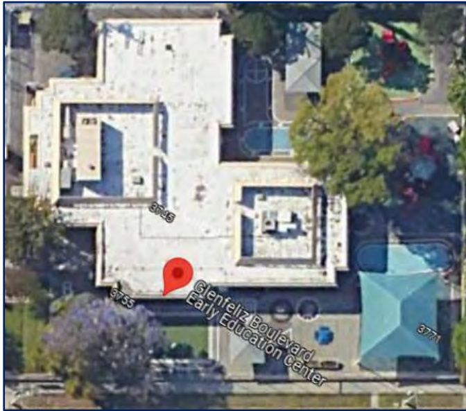
Site Aerial View
