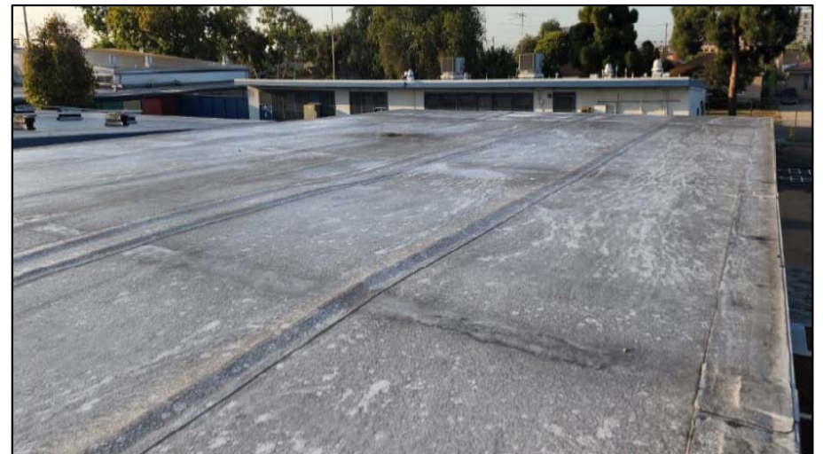
Deteriorated Roofing
