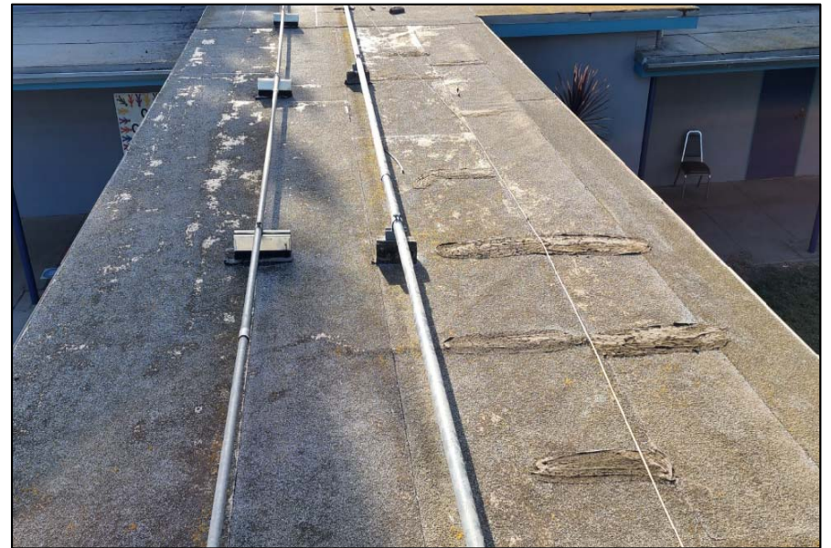
Deteriorated Roofing
