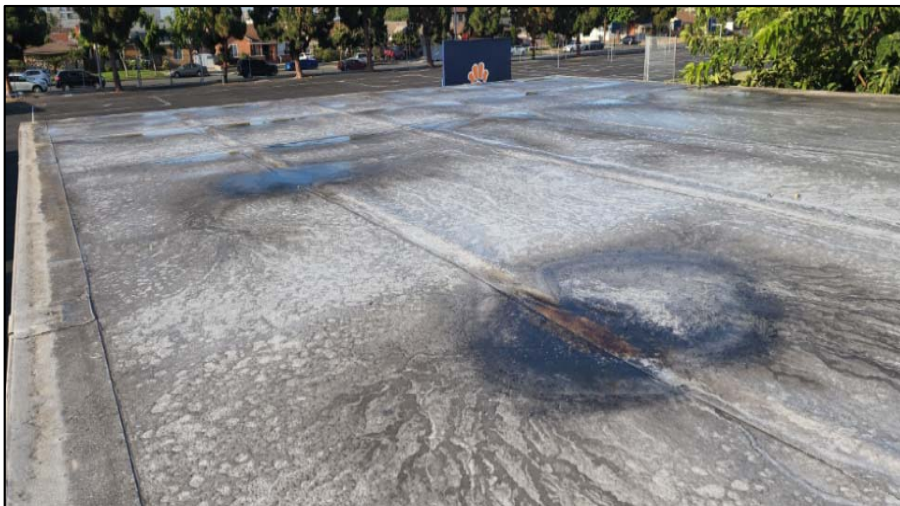
Deteriorated Roofing
