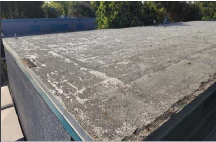
Deteriorated Roofing
