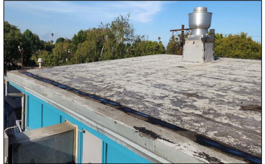
Deteriorated Roofing
