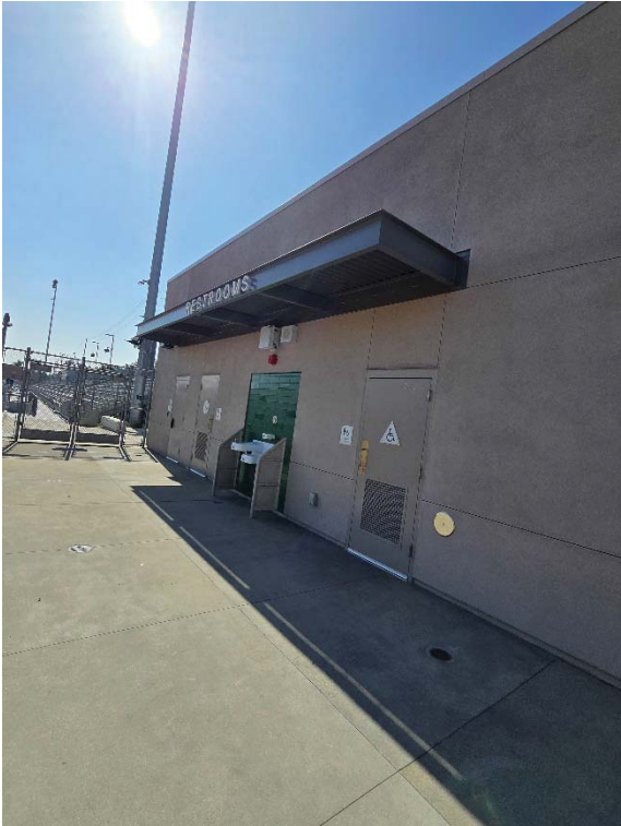
New stadium restroom building
