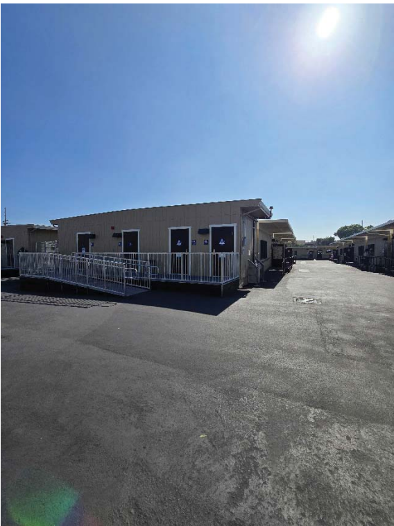
Interim Housing – New restroom building
