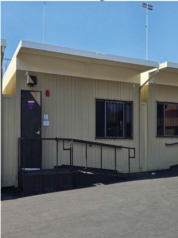
Interim Housing – New classroom building
