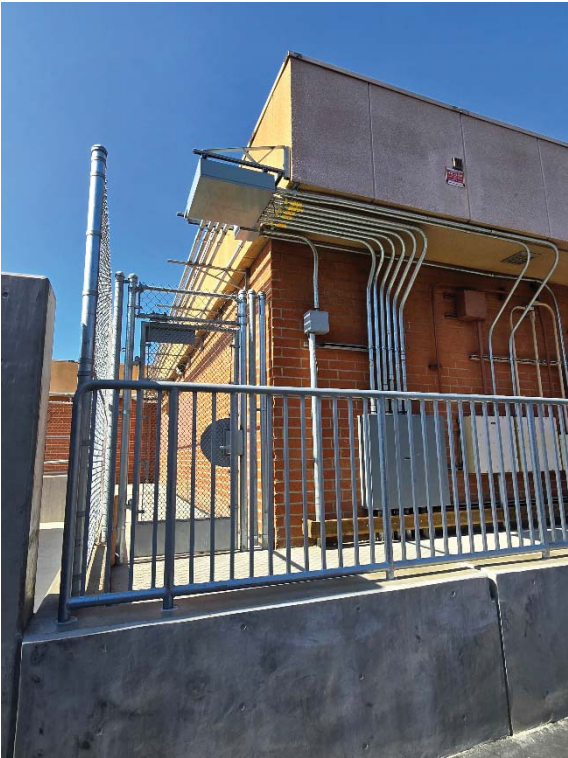
Utility connections related to new LADWP Utility Yard
