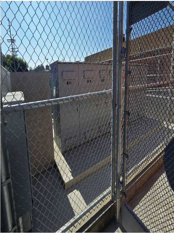
New LADWP Utility Yard - interior
