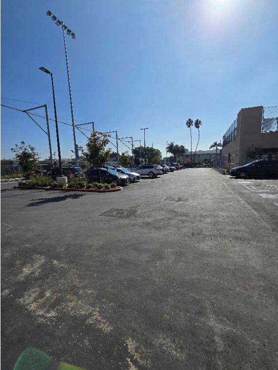
New parking lot adjacent to stadium
