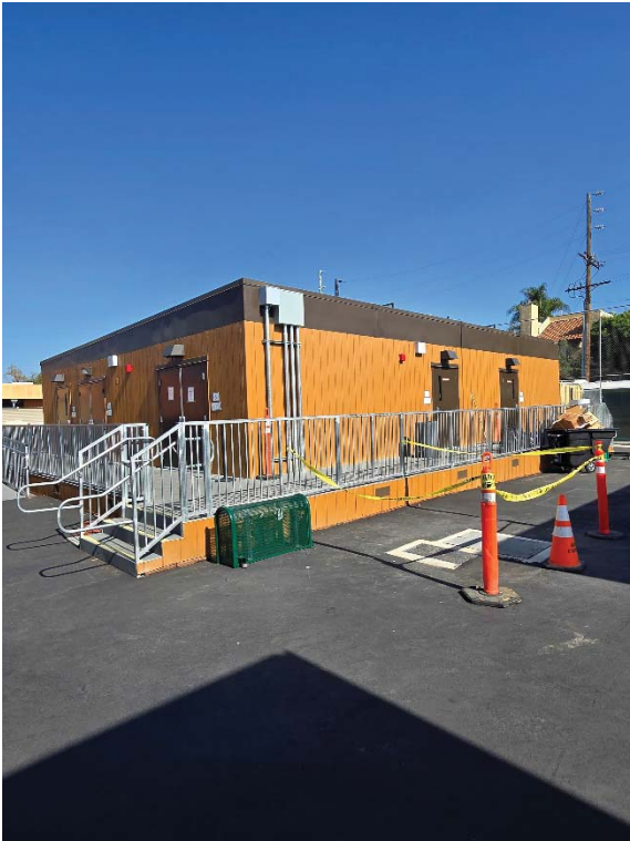
Interim Housing – New kitchen and scramble building
