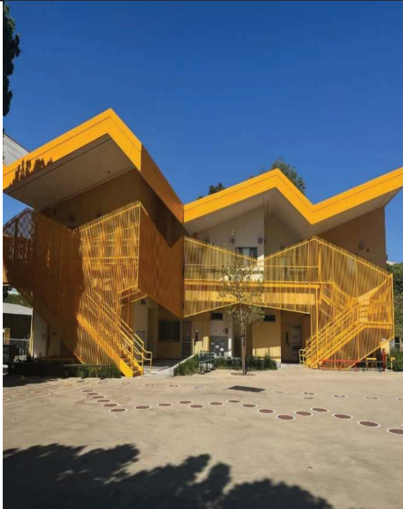
1. Exterior View of New Two-Story Classroom Building
