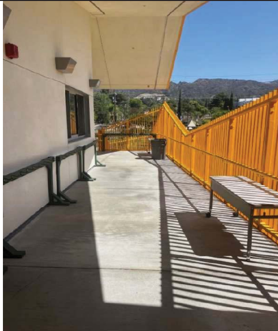
4. 2nd Floor Open-Air Corridor with Protective Yellow Guardrails
