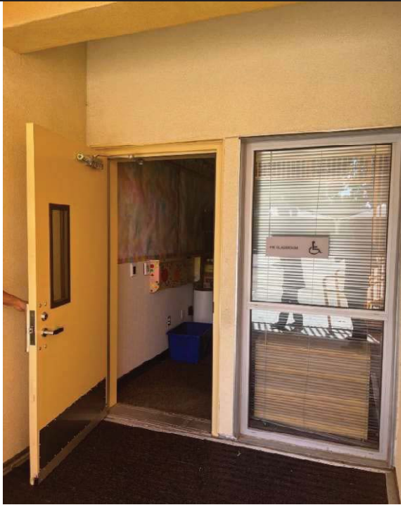
5. 1st Floor Classroom Entry Area
