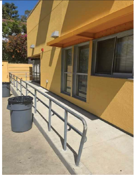
2. ADA-Compliant Handrail and Ramp
