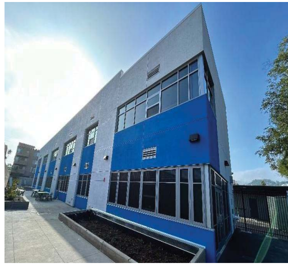
Classroom Exterior – North Elevation
