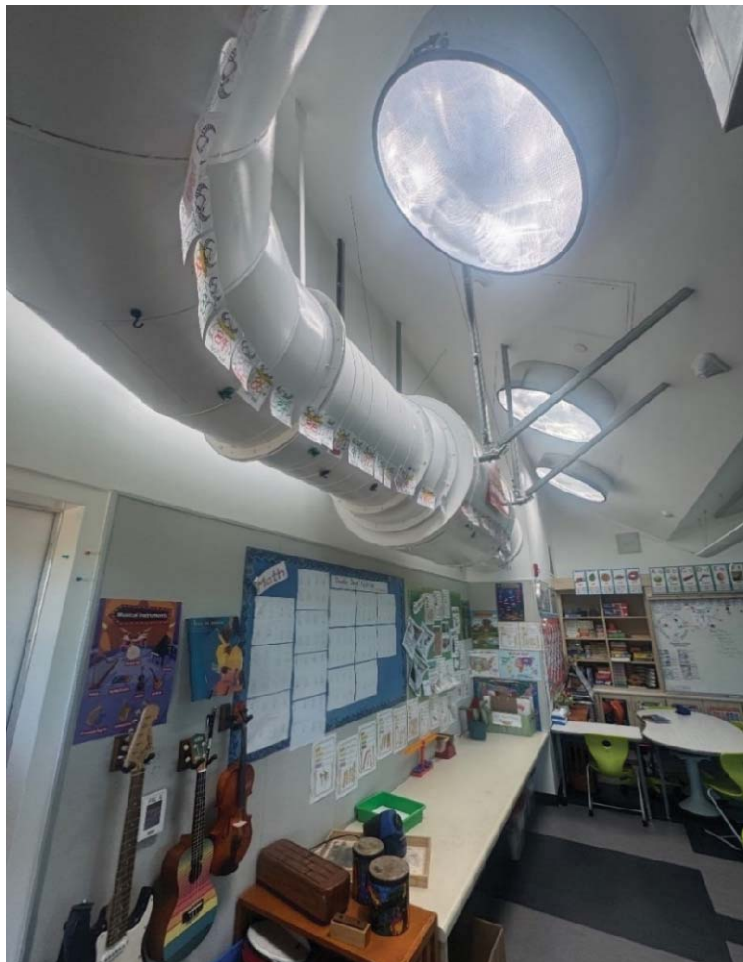
Figure 18. Dahlia Heights ES- View of Duct Silencer at Classroom 3 (OIG Photo - June 25, 2025)
