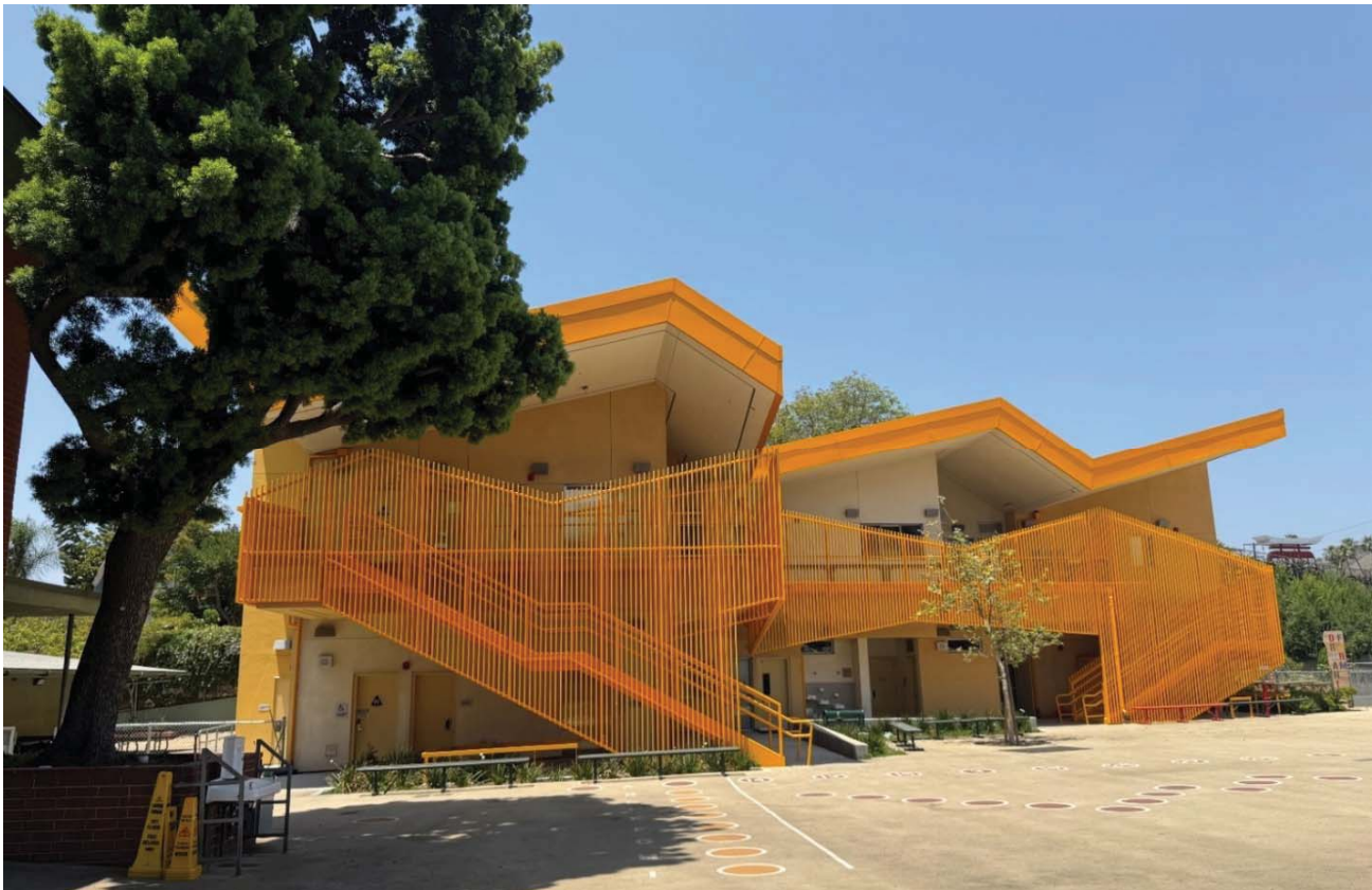
Figure 1. Dahlia Heights ES – Classroom Building Exterior View (OIG Photo- June 6, 2025)
