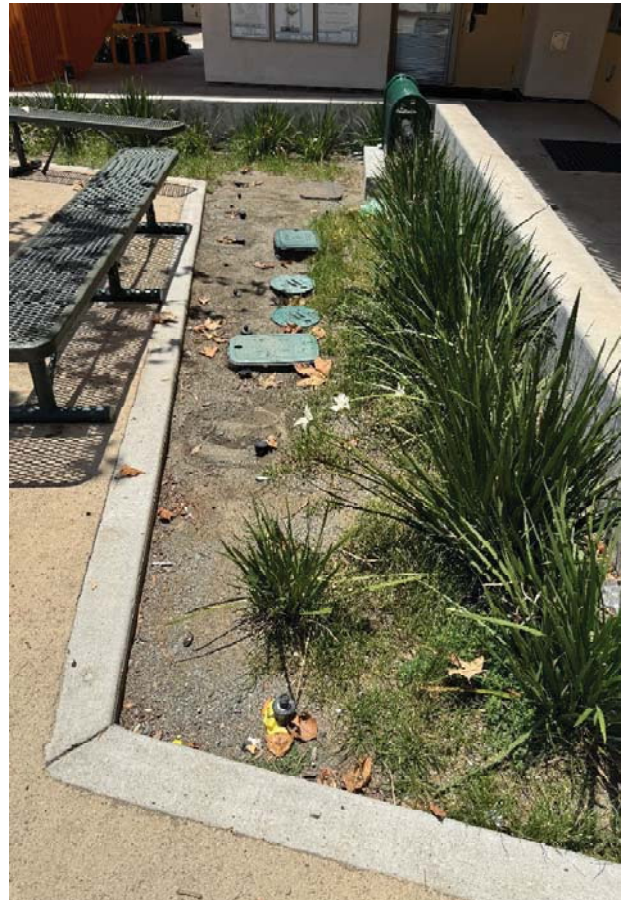
Figure 5b. Dahlia Heights ES Bioswale Garden Feature (OIG Photo-June 25, 2025)
