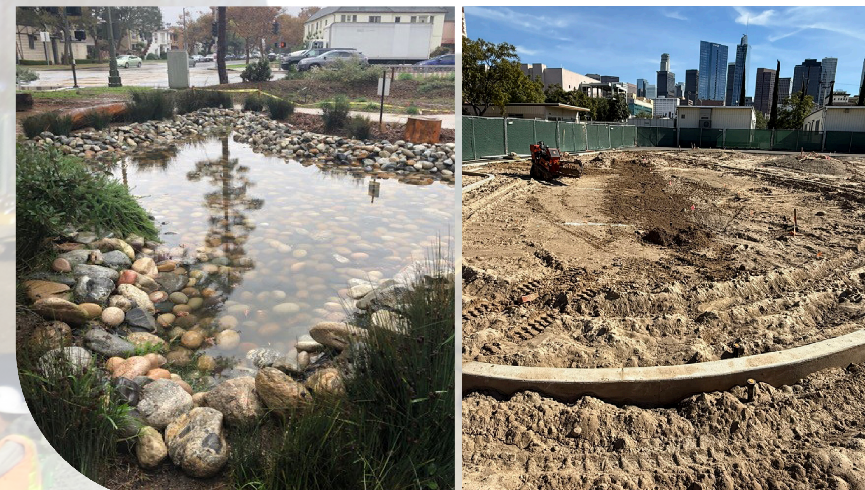
(bottom-left) Infiltration swale at Carthay Environmental Magnet; (bottom-right) Bioswale construction at Esperanza Elementary
