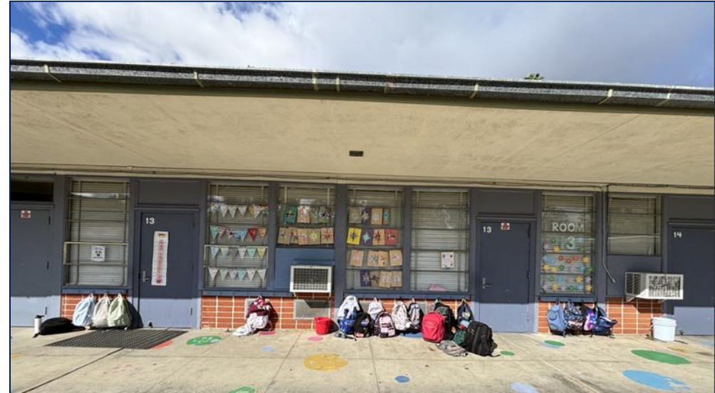
Typical Classroom Building with package wall units
