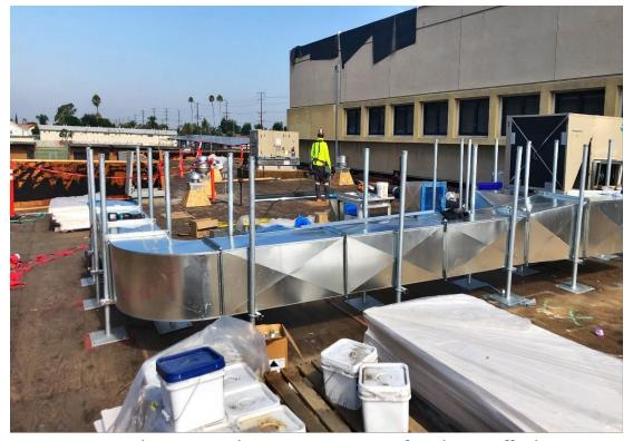
**Gymnasium: Exterior HVAC Duct and Unit Installation**
