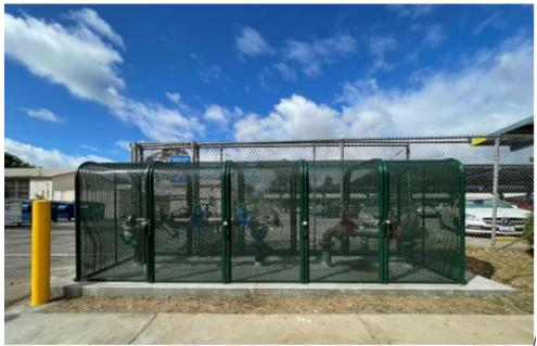
New Backflow Assemblies for Domestic and Fire Main Supplies Installed on 3rd Street
