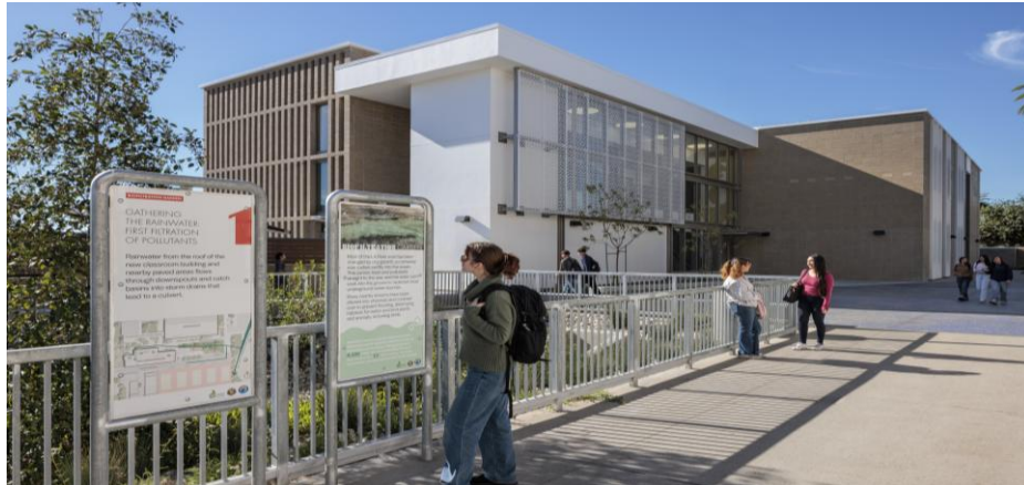
Kennedy HS Comp Mod New Classroom Building
