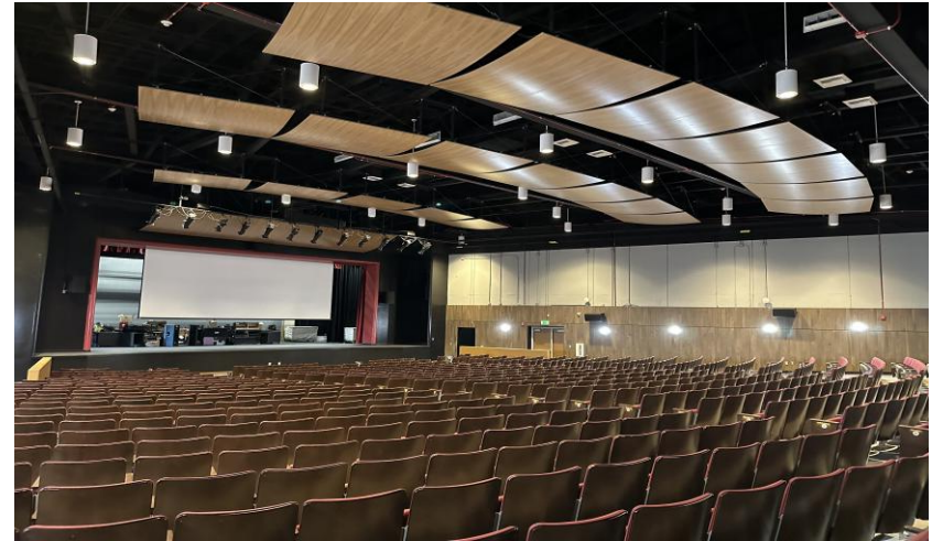
SOCES Comp Mod – Performing Arts Seismic Retrofits Interior
