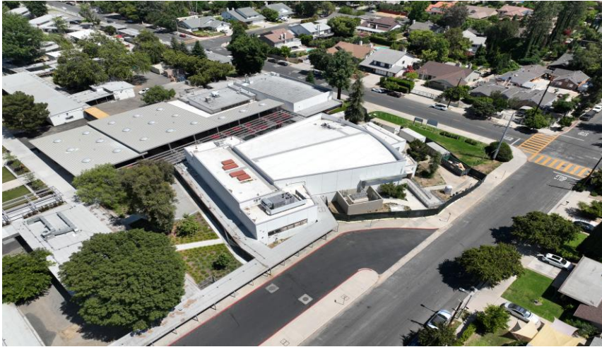
SOCES Comp Mod – Performing Arts Seismic Retrofits Exterior
