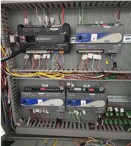
HVAC control panel rework
