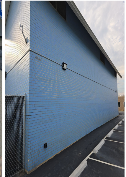
B.6 Lighting upgrades
