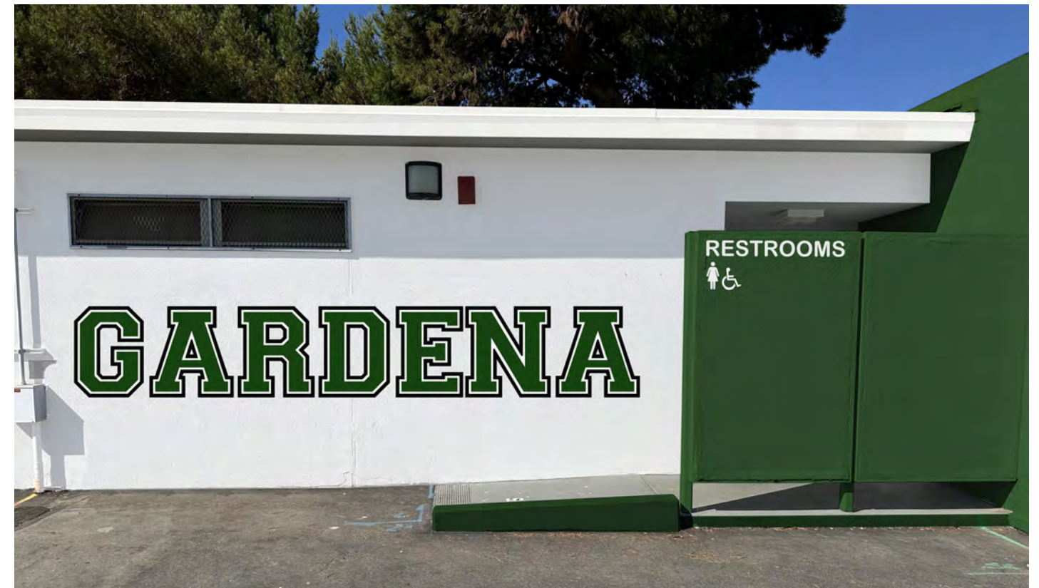
EAST (HOME) AND WEST (VISITOR) FACADE
